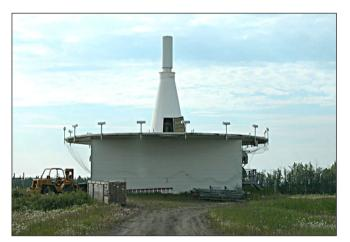
Distance from the beacon is determined by a co-located transponder-based system (Distance Measuring Equipment) using a pulsed-pair signal in the 1000 MHz band.
